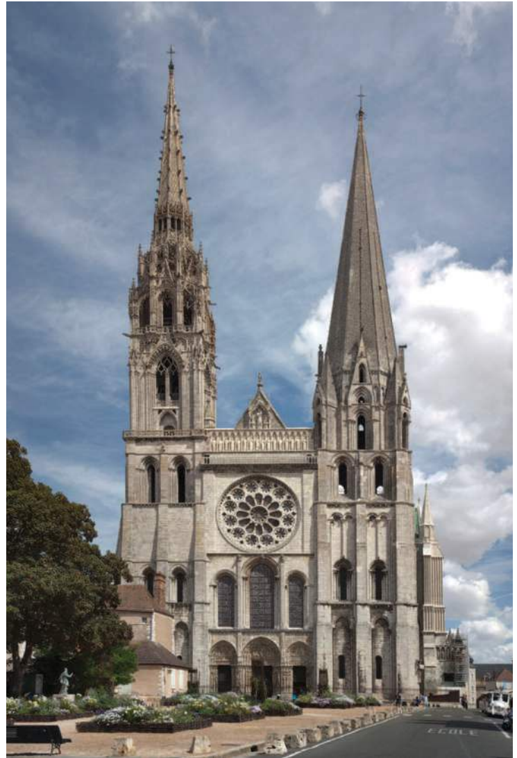
Fig. 17-17 West facade, Chartres Cathedral, France, ca. 1134–1220; south spire, ca. 1160; north spire 1507–13.
