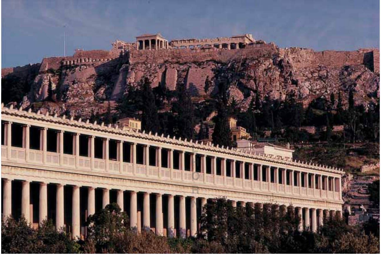
FIGURE 12.5 The Stoa of Attalus in Athens. A roofed colonnade donated to the city of Athens by King Attalus II of Pergamum in the second century BCE, the Stoa (rebuilt in the twentieth century) originally offered shelter for meetings and discussions, such as the debates with Athenian philosophers that Paul is said to have held when he first visited Athens (Acts 17). The Acropolis rises in the background.
