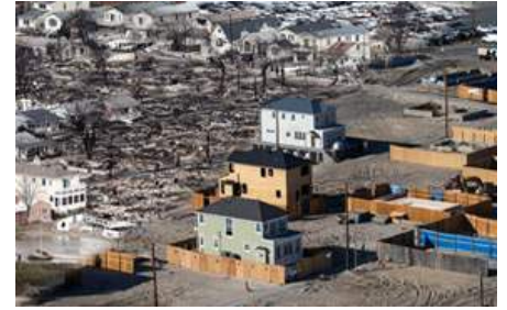
Hurricane Sandy, Before and After, One Year Later
