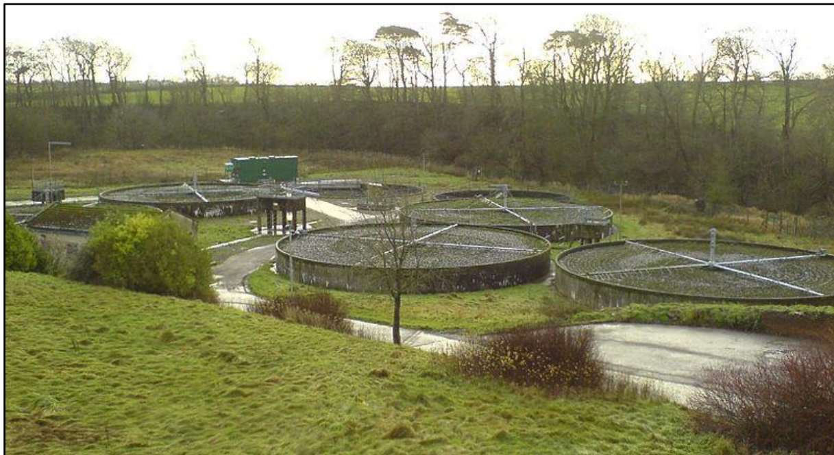
Wastewater treatment works in Ayrshire, Scotland. (Qualit-E, 2009)
